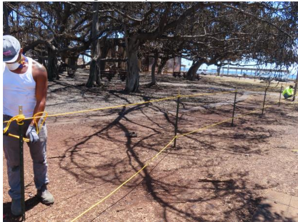
Establishing a tree protection zone
